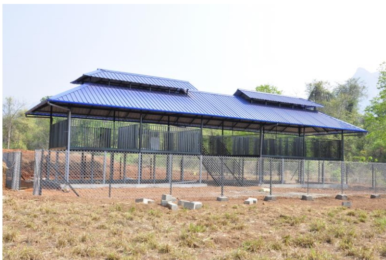
Newly constructed goat shed
