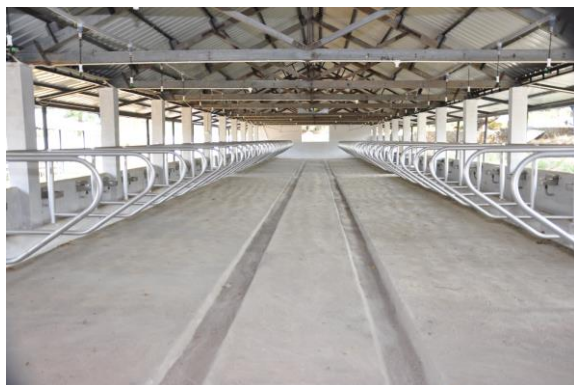
Renovation of cattle shed
