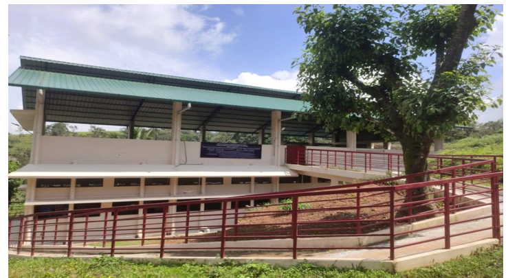
Fig. Two storey pig sty with ramp
