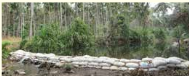
Water self sufficiency campaign - Construction of temporary check dams
