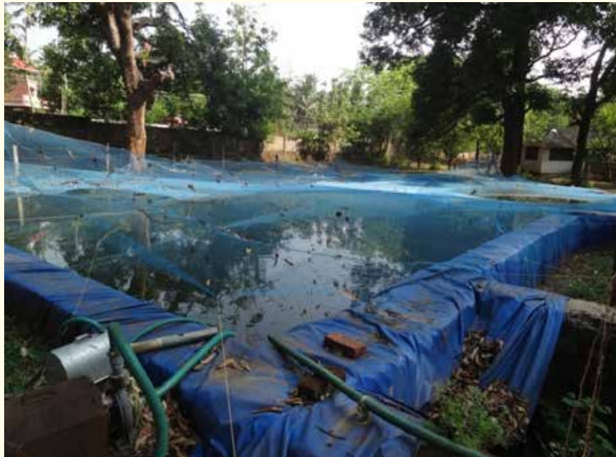
Rain water harvesting tank
