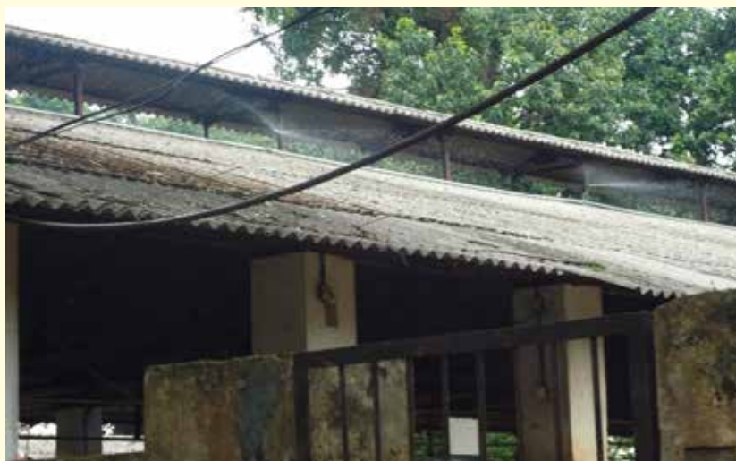
Roof top sprinklers
