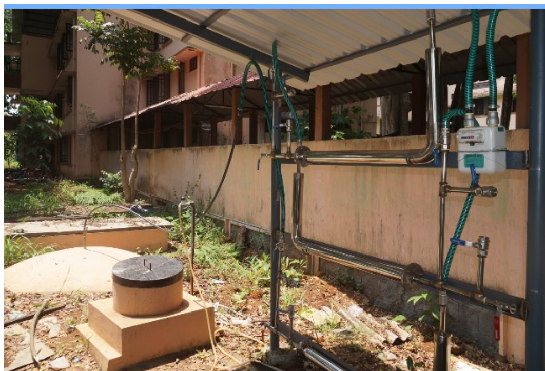
Biogas Plant and Scrubbing unit established at Mannuthy campus
