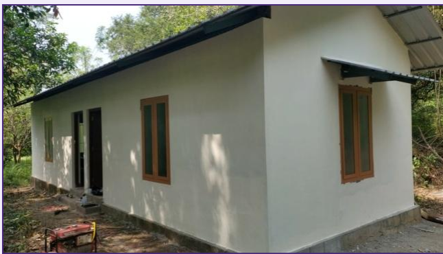
Hill top comfort station and waiting rooms for farm labourers at fodder production area
